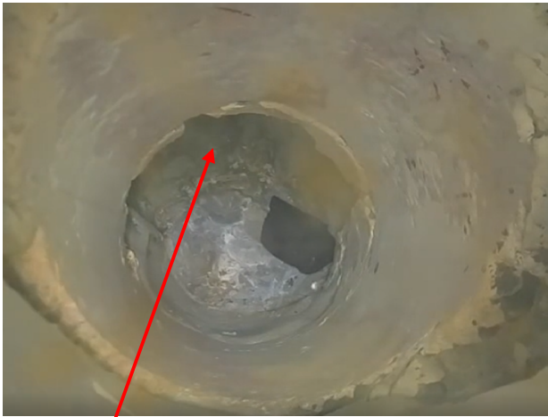
View from RGeo-eye® showing a missing section of the borehole wall.
